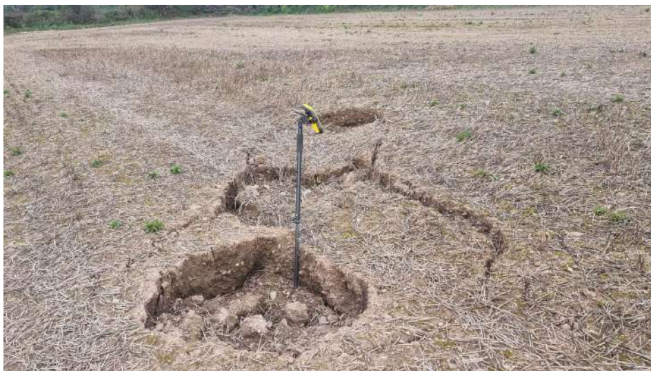
Figure 2.1D. Subsidence feature in south of site.
